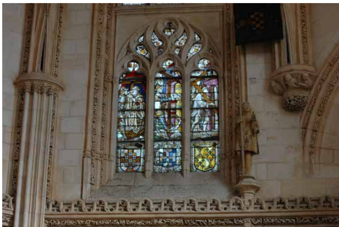
Fig. 9.12 Simón de Colonia, Chapel of the Condestable, Burgos Cathedral (1480/90s).
